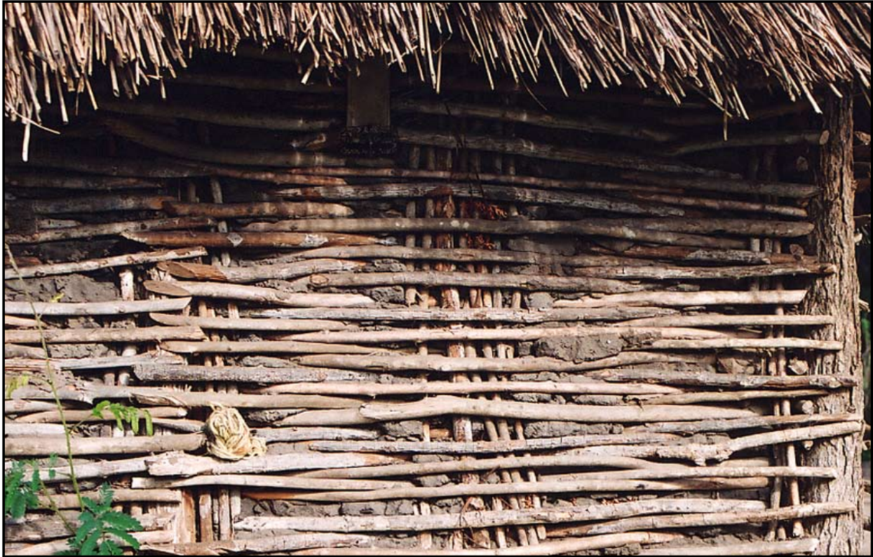
Figure 4. A typical wooden wall made from interlocked woven wooden laths laced between main support posts in the community of Manqakulane, Maputaland, KwaZulu-Natal province, South Africa, as established by a survey in 2002.
