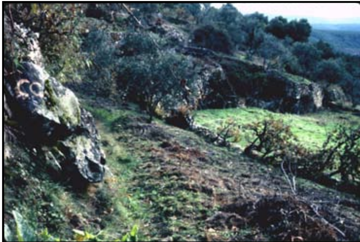
Figure 2. Contoured terraces in Val Pasqual; between curving soil retaining walls and a thick grass strip runs an irrigation ditch evident in the lower left; the continuing grass strip is visible right center as darker green at the base of the wall.
