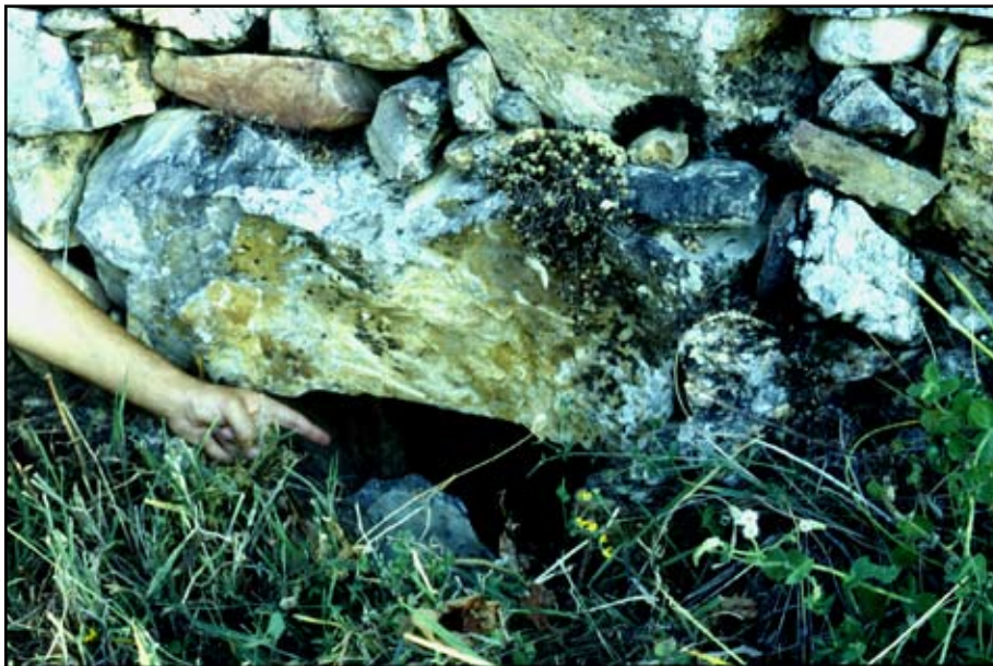
Figure 6. Larger quartzite rock near base of soil retaining wall serves as lintel to allow irrigation water that has filtered through the soil of the terrace above and collected against the bed rock to emerge at the top of the terrace below to reuse for irrigation.
