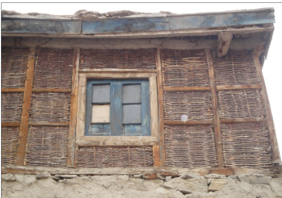
Fig. 3. A typical house with woven walls (shaq nang)
