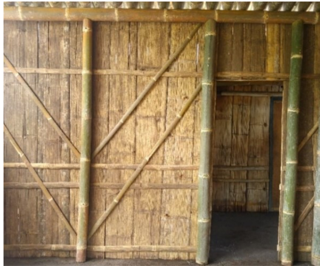
Figure 7. Application of naja , tubo , and lat in the house wall in Ratogesa Village.
