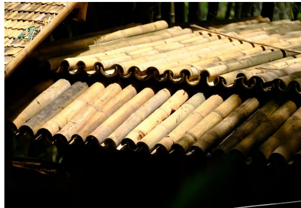
Figure 9. Application of lenga from the outside in Wogo Village.
