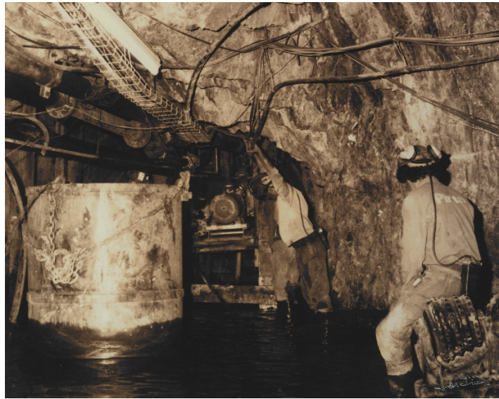
Figure 8. Water table inside the mine. © Luís Matias and Aljustrel Municipality.
